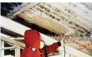
**Figure 7.5** Shadow vacuuming during unscrewing of board
