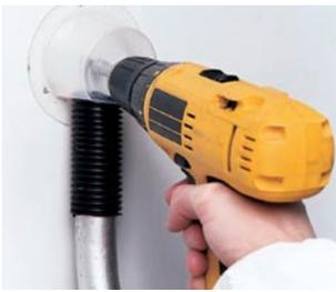
**Figure 7.7** Textured coating being drilled through paste
